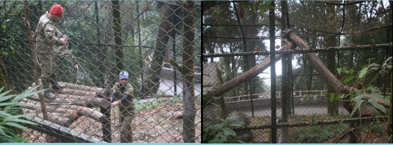
New resting platforms and new aerial walkways in the carnivore enclosures
